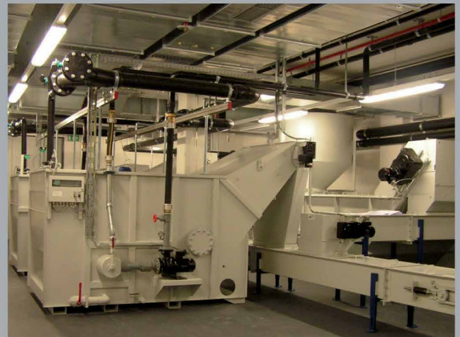
Central system for 3.000 lpm grinding emulsion
